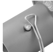
Fig 3 Improperly Secured Leg Coupling Pin
